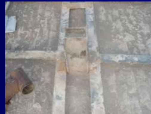
Steel I-beams with flat arch and bracing steel bars
