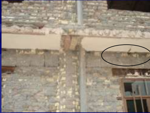
Steel I beam as lintel above window opening
