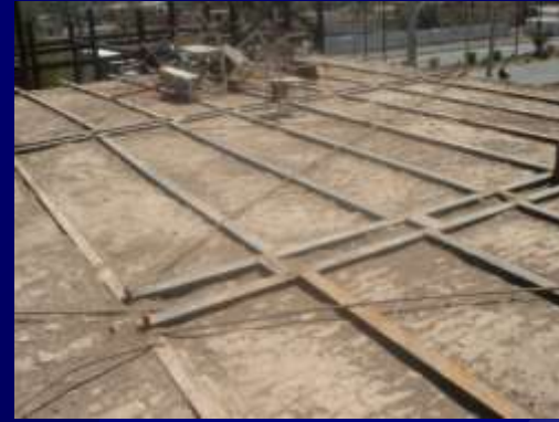
Steel I-beams with flat arch and bracing steel bars
