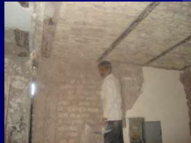
RC column, RC bond beam, flat arch and expansion joint
