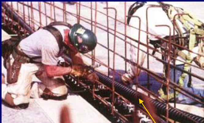
Post tensioning under progress Conduit
