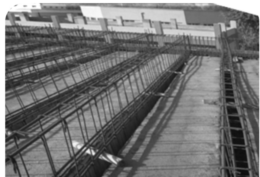
Beam Reinforcement
