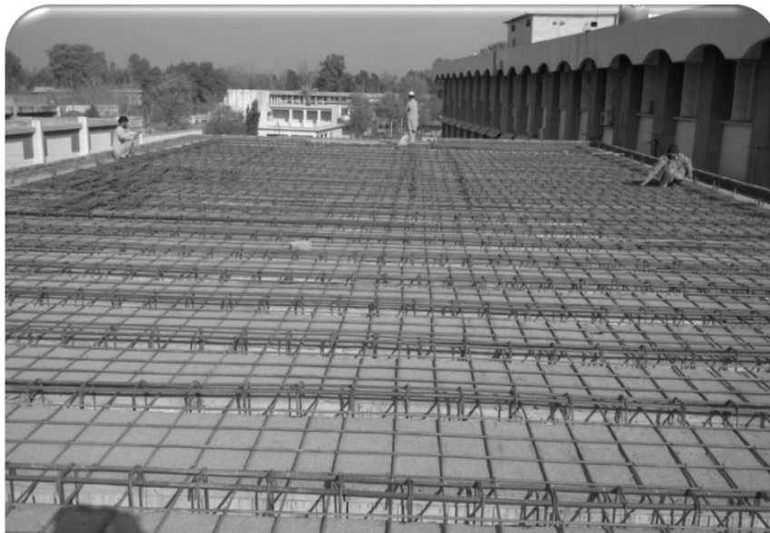
Slab Reinforcement
