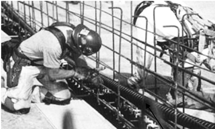
Post tensioning under progress Conduit
