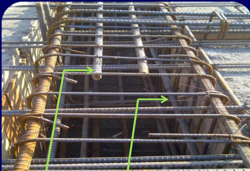
Curtailed and Skin Reinforcement
