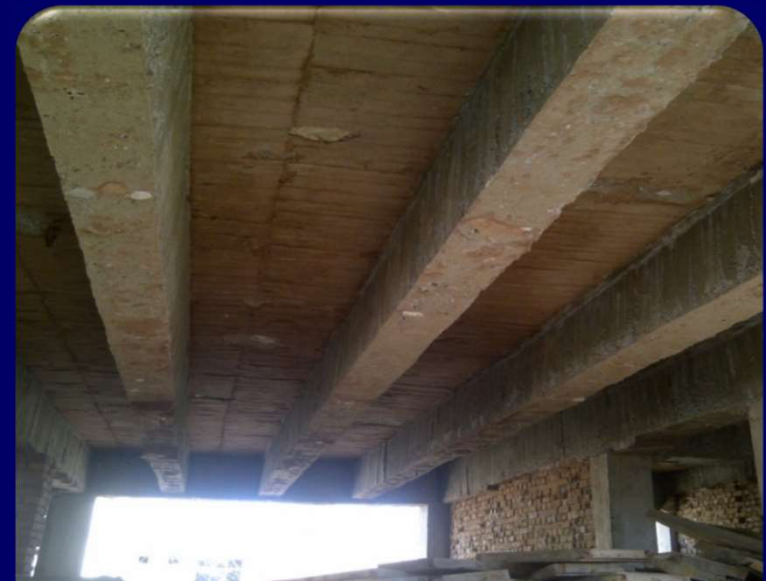
Hall after completion
