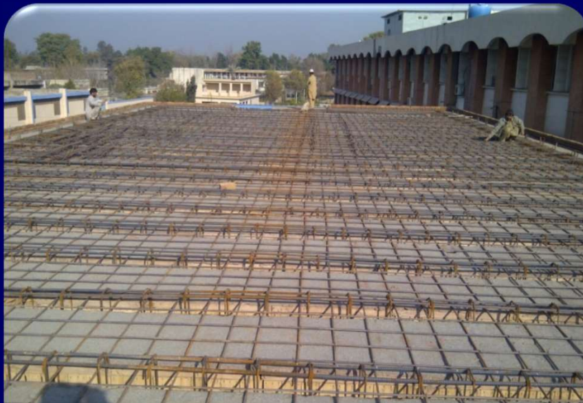
Slab Reinforcement
