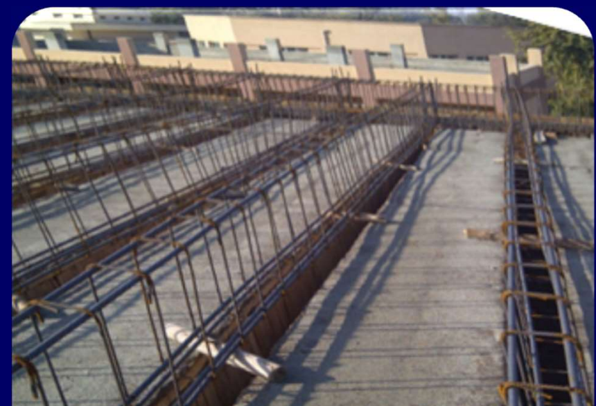
Beam Reinforcement
