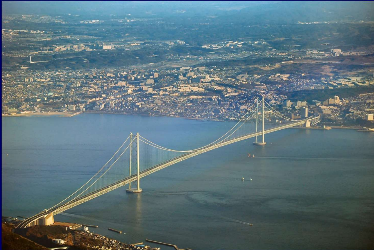
Akashi Kaikyō Bridge, Japan (1991 m)
