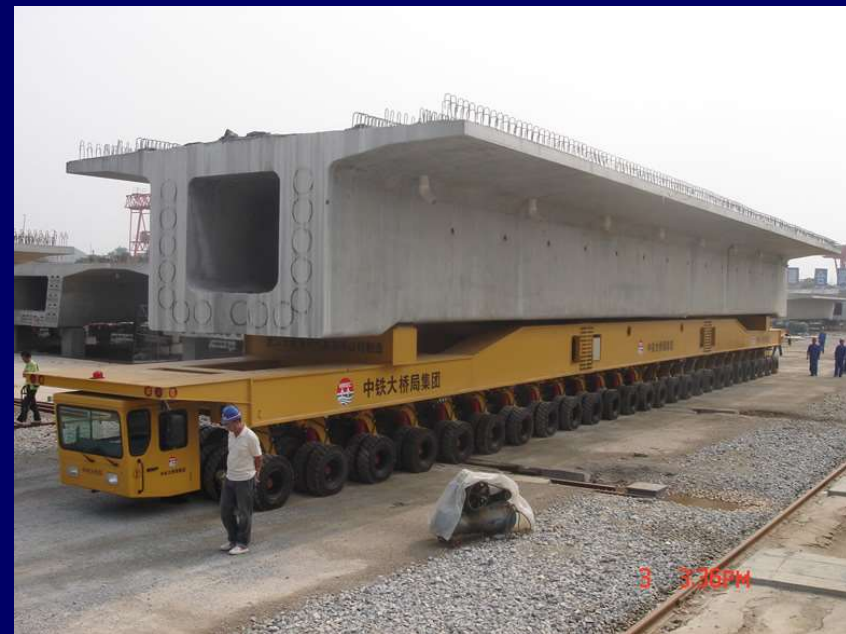
Concrete Box Girder Bridge
