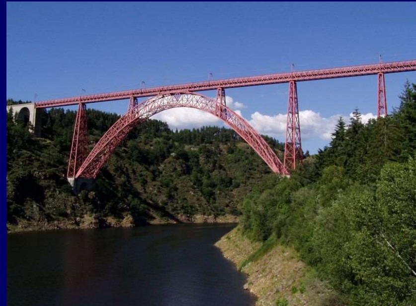
Steel Truss Arch
