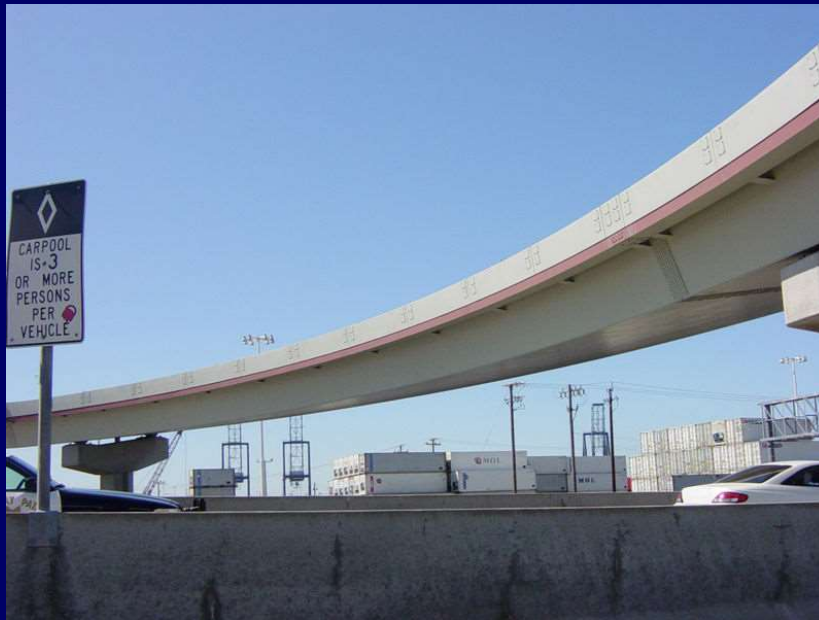
Box Girder Bridge
