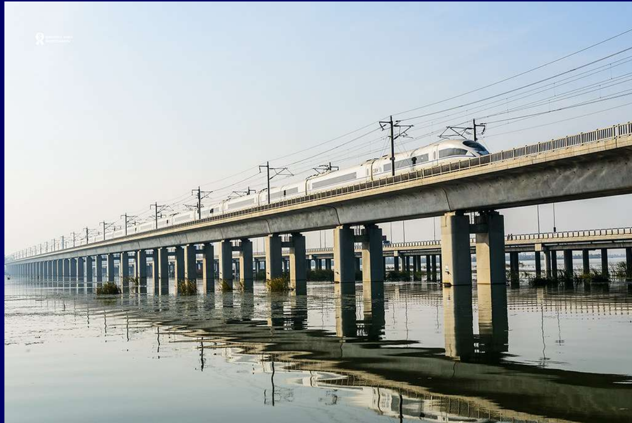
Danyang–Kunshan Grand Bridge in China (164800 m)
