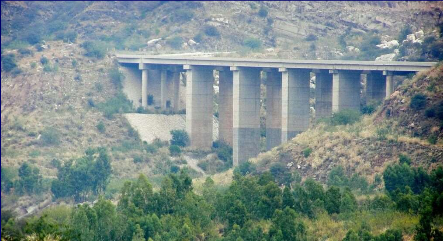
Bridge at Kallar Kahar, M2 Motorway
