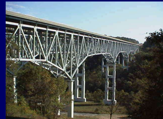
Steel Deck Truss Bridge
