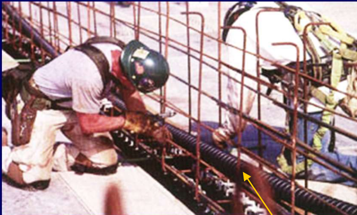
Post tensioning under progress Conduit
