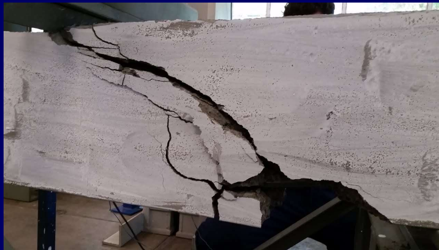
Rupture (Flexure, shear or combination )
