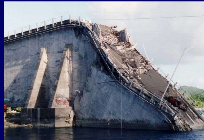
Fatigue (Failure due to repetitive cyclic loading)
