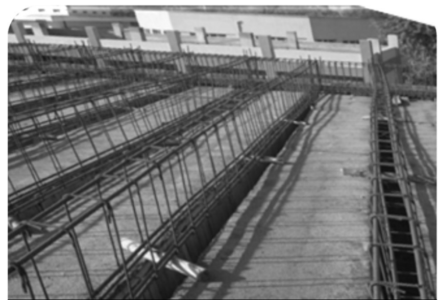
Beam Reinforcement
