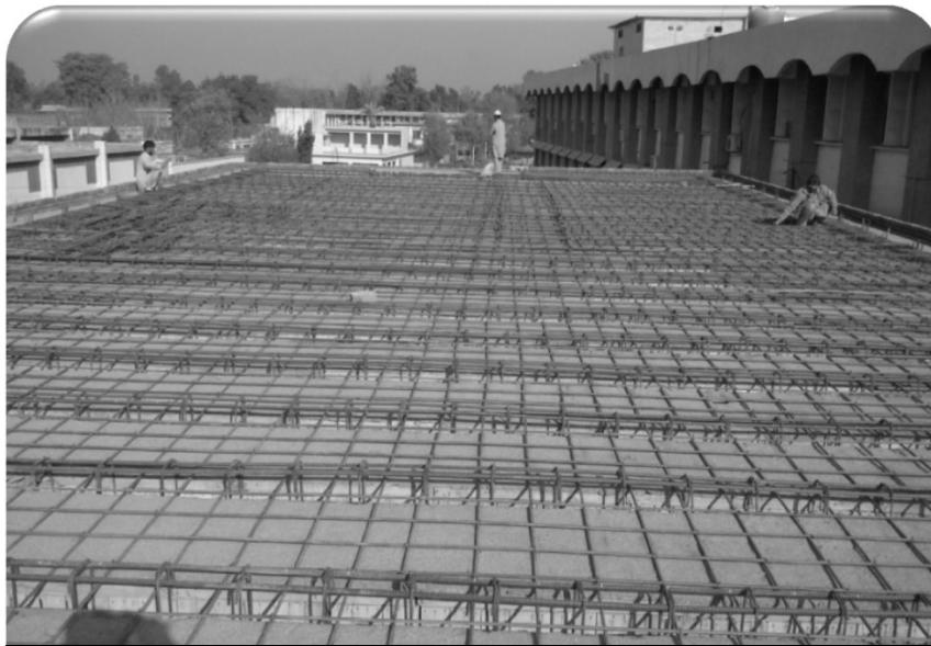
Slab Reinforcement
