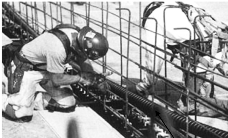
Post tensioning under progress Conduit
