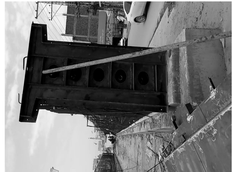
Post-tensioned Concrete Girder at BRT Peshawar (video clip)
