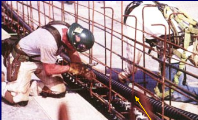
Post tensioning under progress
